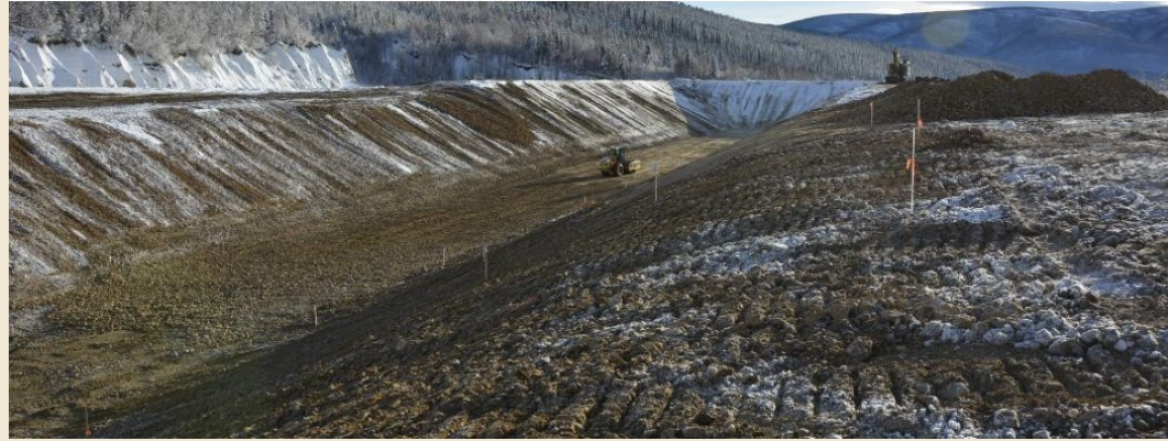
Repair of IROSA 2, October 2025
