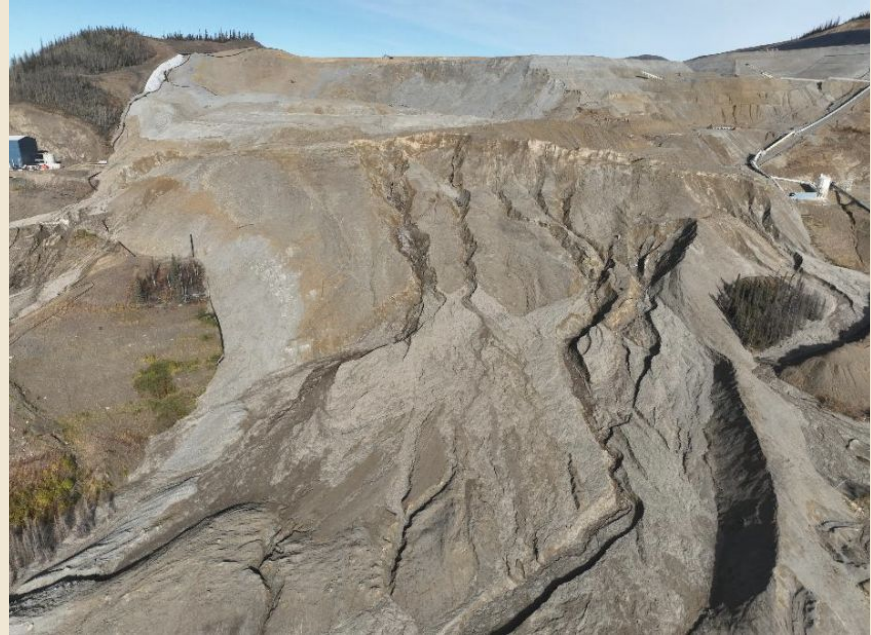
Heap Leach Facility Oct 2, 2025
