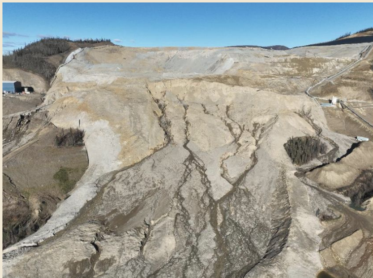
Heap Leach Facility Oct 2, 2024
