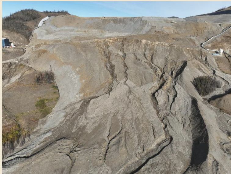
Heap Leach Facility Oct 2, 2025
