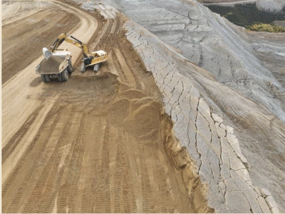
Excavating material above failure scarp, Sept. 15
