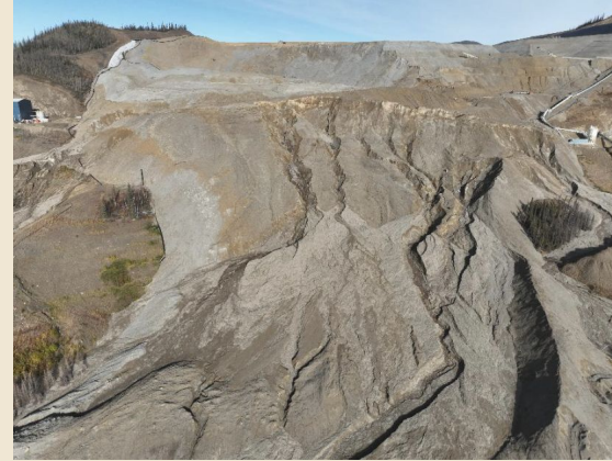
Placing material at back of HLF, Sept. 15
